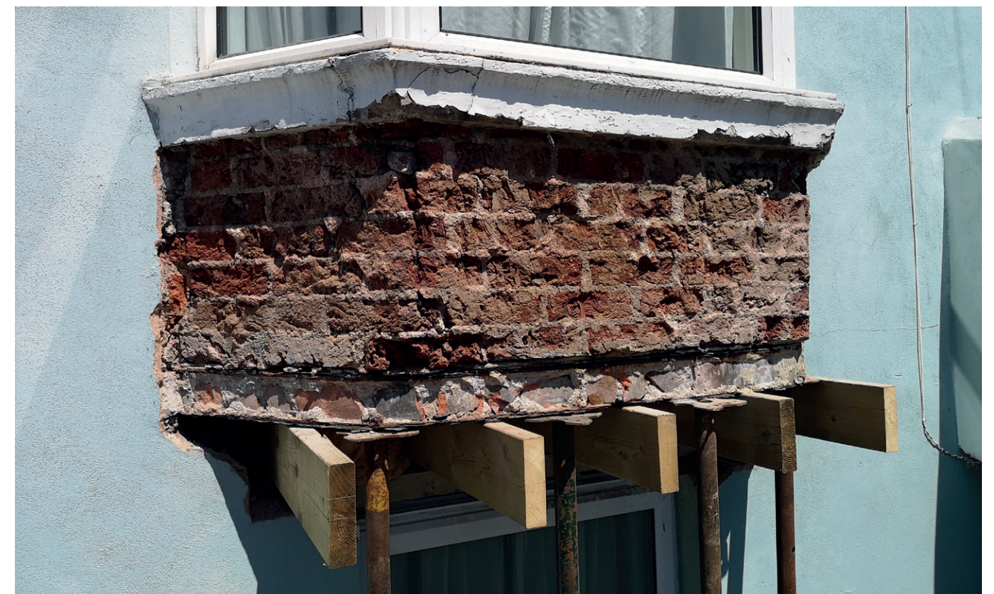
Photo 2 shows the beam, new bay supports and the Acrow props.
