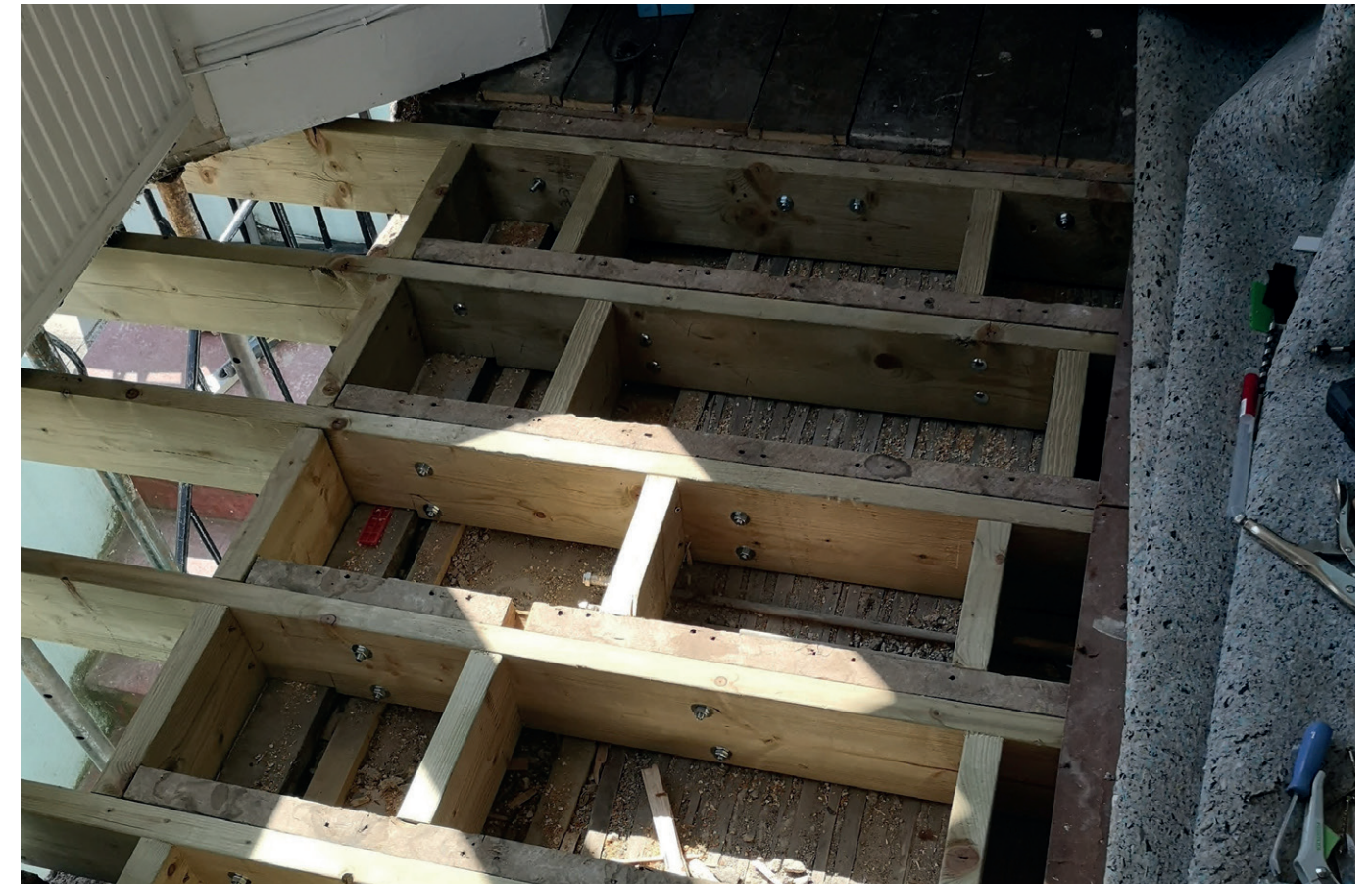
Photo 2 shows the beam, new bay supports and the Acrow props.
